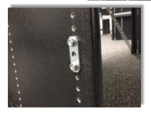
3. Tighten nuts down onto backing plate.
